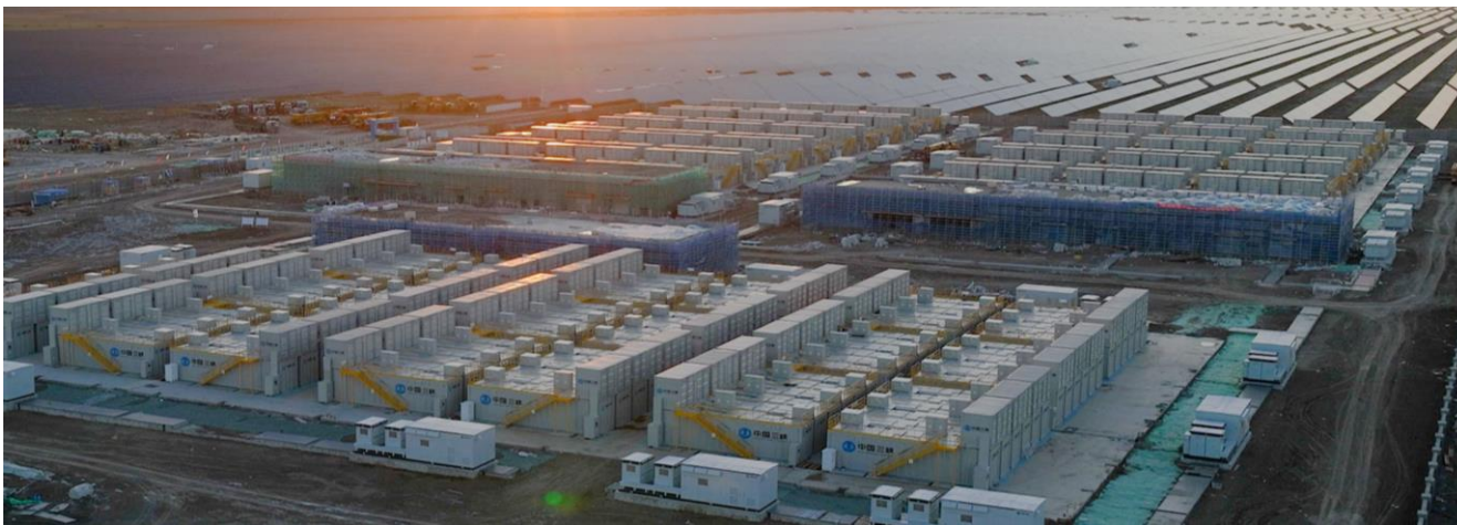
Source: RKP Global— Jimusaer/Xinjiang VRFB Project, China200MW / 1GWh VFB VBESS Utility-scale long-duration storage deployment supporting renewable integration and grid stability
